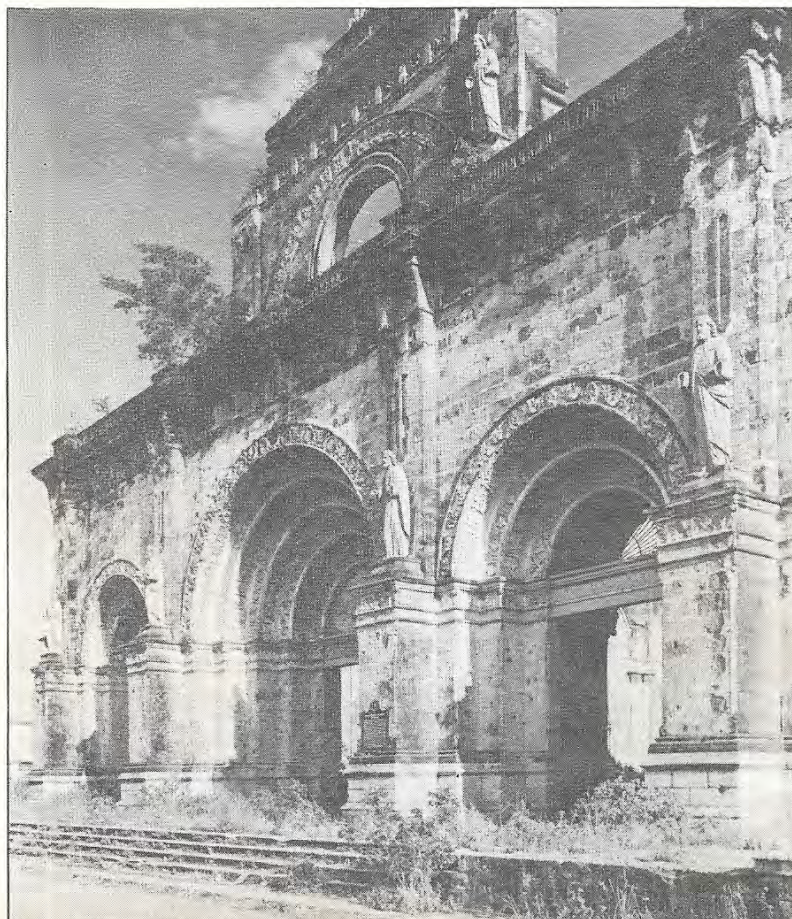
THE BEAUTIFUL PAOAY CHURCH IN ILOCOS NORTE. BUTRESSES ARE FOR PROTECTION AGAINST EARTHQUAKES.
